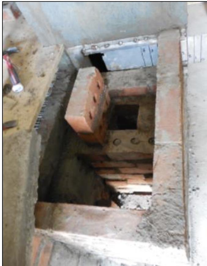
Figure 14 Top of the flame tunnel
