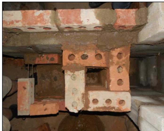
Figure 19 Increased vertical flame tunnel
