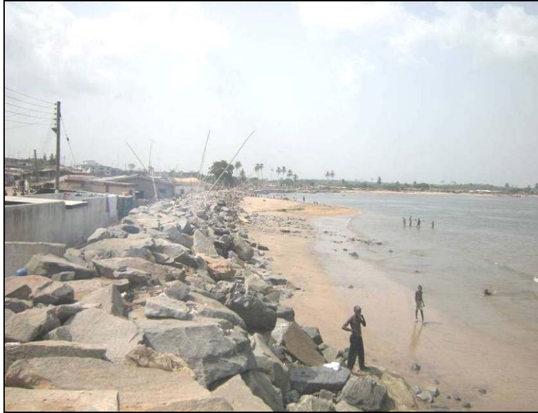
Figure 14: Eroded Beach in Shama District
