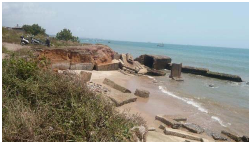
Figure 15: Coastal Erosion on some beaches in the Western Region
