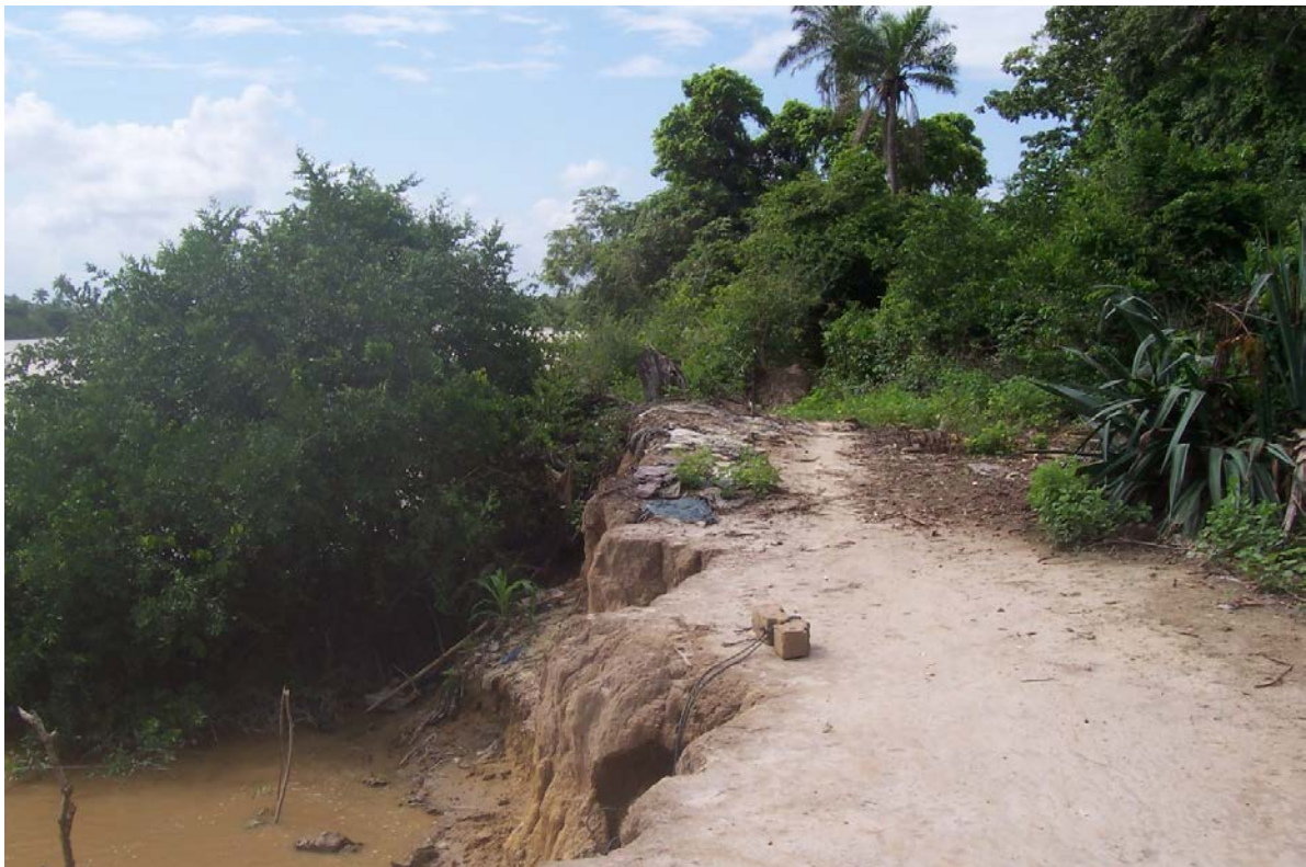
Plate 15i: Effects of Erosion at Krobo
