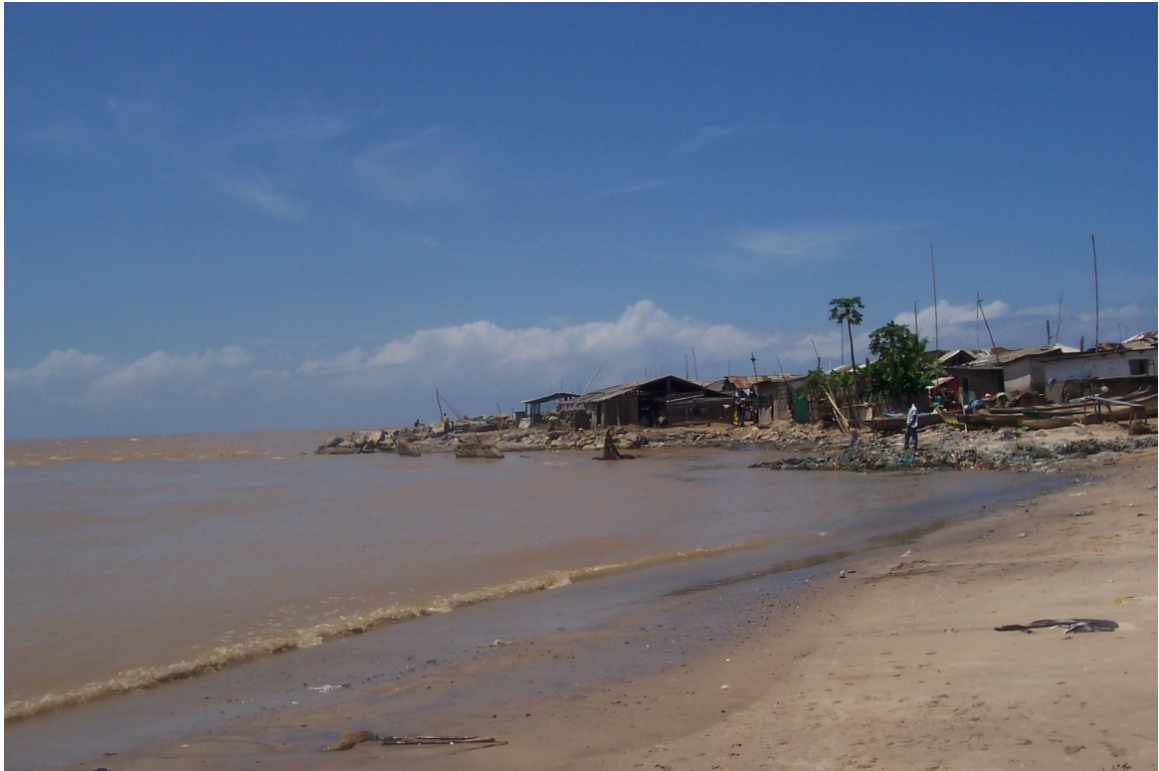
Plate 7 ii: Shama Sea Defence Wall
