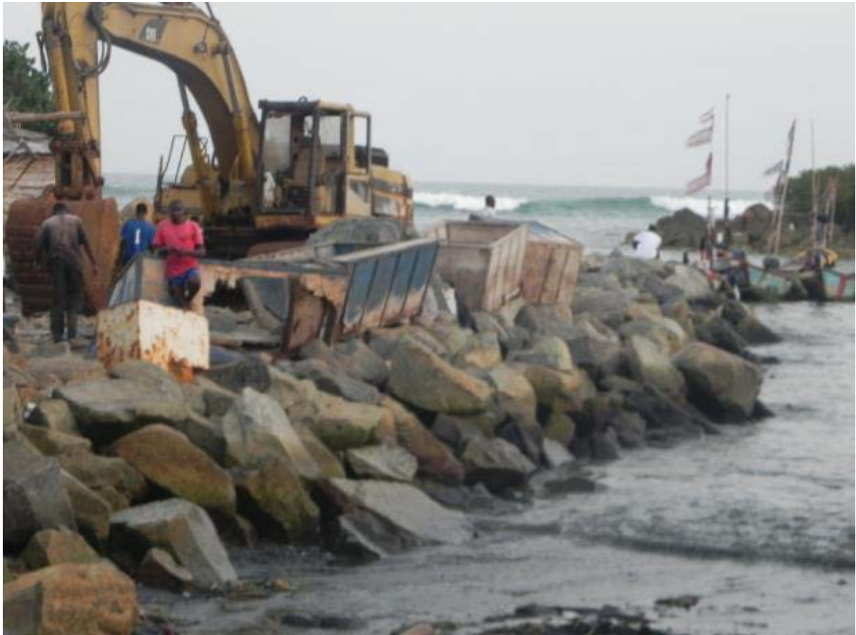
Figure 20 Incomplete and damaged harbor defense system in Ahanta West is evidence of past attempts to protect the harbor and ongoing damage from high wave energy
