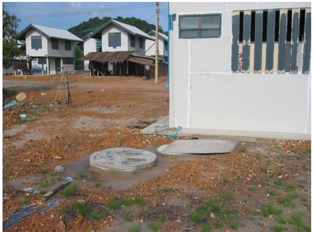
Figure 10. Toilet system at Village No. 7
