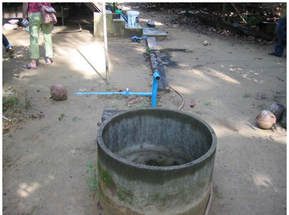
Figure 2. Typical shallow well in a village
