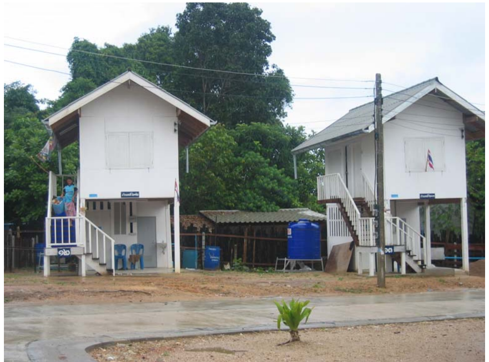
Figure 5. A 1.5 m 3 plastic tank for rainwater collection
