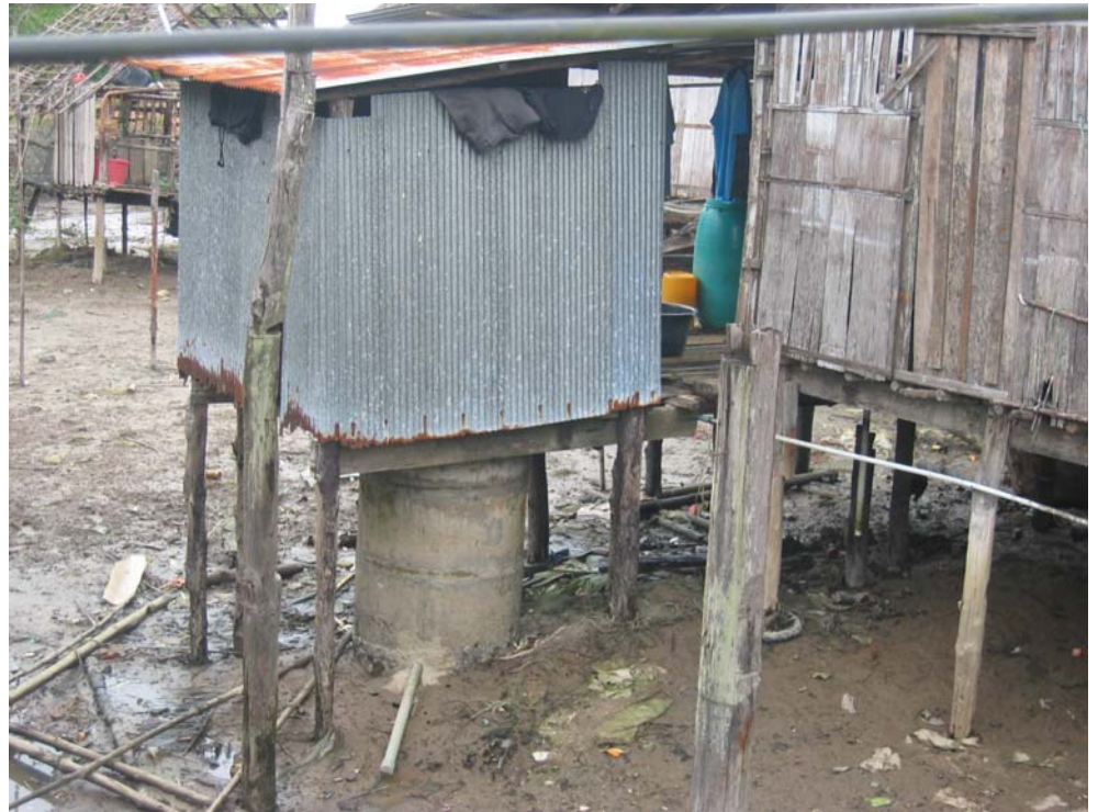
Figure 9. Toilet system at Village No. 4
