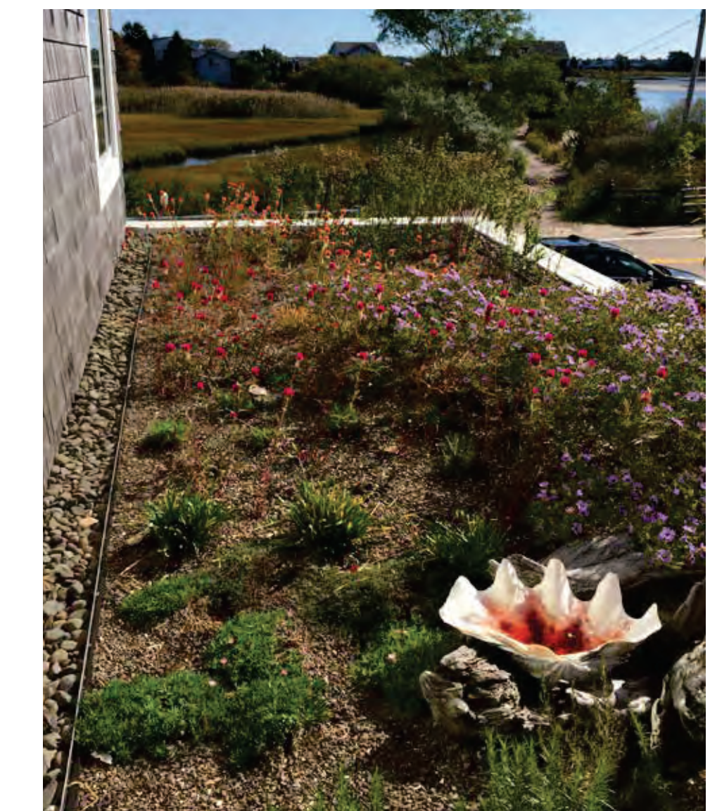
Green Roof Infrastructure Green roofs are an effective way to capture stormwater runoff and beautify Wickford.
