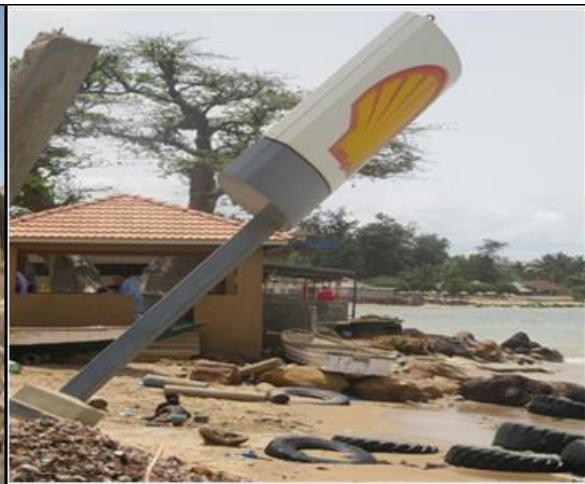
Photo 32: Gas station at risk of coastal erosion in Saly
