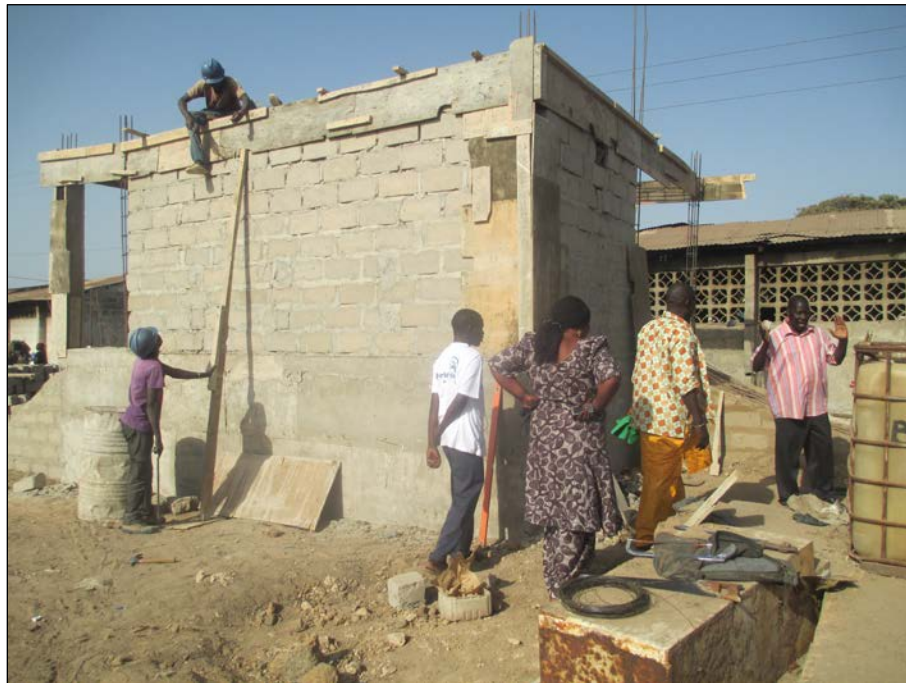
Figure 16. Progress on construction of the Tanji fish landing site toilet facility as of March 26th.
