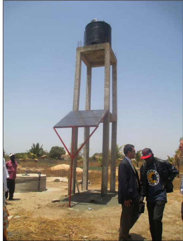
Figures 13 and 14. (from left behind the tap) The U.S. Embassy Charge d’Affairs, the President of the Kartong Fish landing site WASH Committee (the woman) and the CEO of GAMWORKS test the new water point. Solar powered pumping and storage system for the protected well that supplies the water point located 500 meters away.
