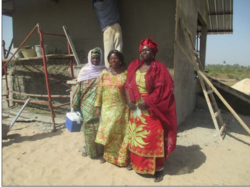
Figure 17. Members of the Sanyang fish landing site WASH Management Committee in front of the nearly completed toilet facility.
