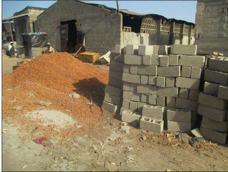
Figure 15. At left, washed laterite used in place of basalt stones for the concrete mixture due to border closures cutting off the basalt supply from Senegal.
