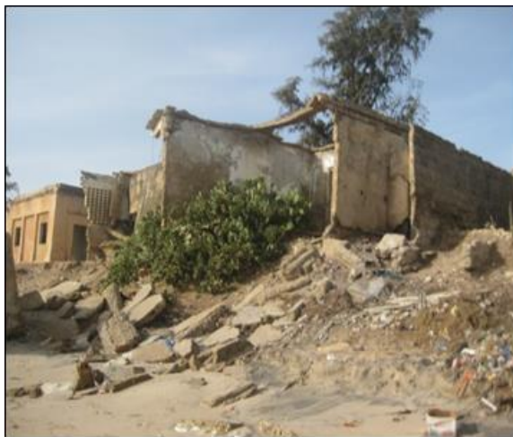
Photo 31: Old building engulfed by the sea in Nianing
