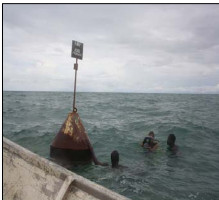
Photo 16: Locating and cleaning a buoy
