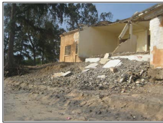
Photo 19: Coastal erosion caused by climate change
