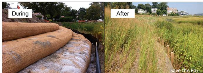
A small park in Cranston features a **regraded and stabilized shoreline** to dissipate wave energy and slow erosion.
