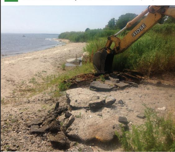
Eroding pavement on the beach was removed, the road was carved back 75 feet and a filter strip was installed to slow and treat stormwater runoff.
