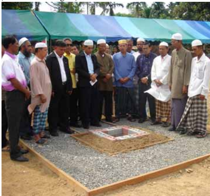
Mr. Songsak Manchit, Islam Chairman of Ranong Province (7 th from the left), leads the religious ceremony for the groundbreaking.
