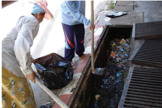
Villagers in Khampuan clean out the community sewer line.
