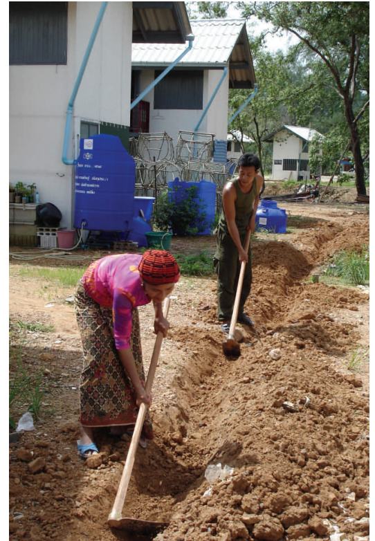
Villagers dig trenches for water pipes in Hat Prapat, Village 2
