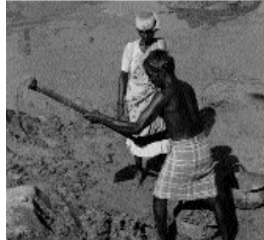
Excavation of shrimp pond in Potential Acid Sulphate Soils (PASS) in Kumta, Karnataka, India (Photo courtesy of Jesmond Sammut, University of New South Wales, Sydney)
